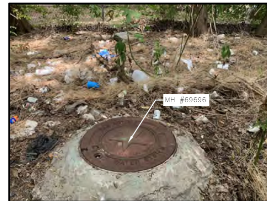
FIGURE 1: DEBRIS NEAR MH #69696 (FACING NORTHWEST).
