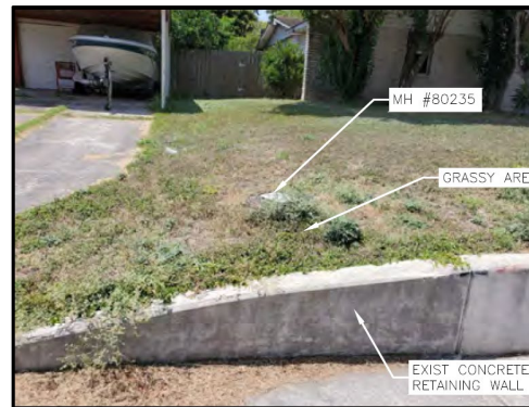
FIGURE 1: EXIST RETAINING WALL TO BE PROTECTED NEAR MH #80235 (NSPI).
