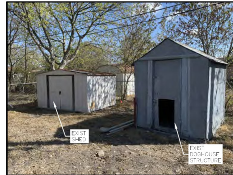
FIGURE 1. EXISTING SHED AND DOGHOUSE STRUCTURE AT 1902 CANTEEN.
